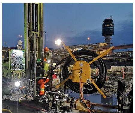
The Memorandum of Understanding between PPI and IGSHPA will advance the benefits that both organizations provide to the geothermal exchange industry. This geothermal system at Vancouver International Airport (YVR) used 841 single U-bend geothermal loops, each 1,000 feet long, with a molded and heat-fused U-bend installed at the mid-point. Image Courtesy Versaprofiles
